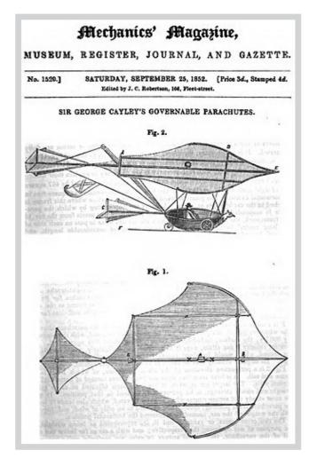
Modern aerospace began with Sir George Cayley in 1799. Cayley proposed an aircraft with a 'fixed wing and a horizontal and vertical tail', defining characteristics of the modern airplane.
