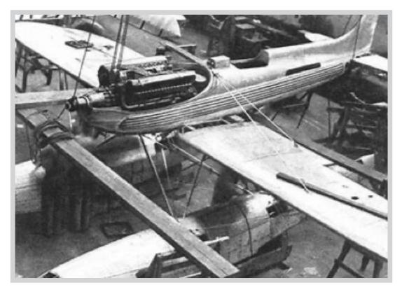
Supermarine S6B showing the new Rolls-Royce R engine.
